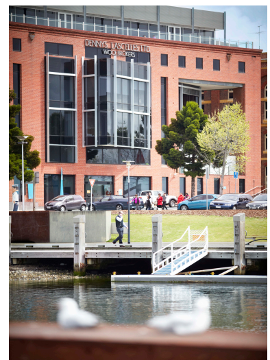
1 Gheringhap Street Geelong Victoria 3220
