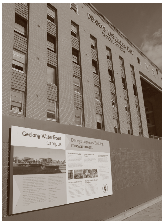
Redevelopment of the Denny's Lascelles building at the Geelong Waterfront Campus has begun
