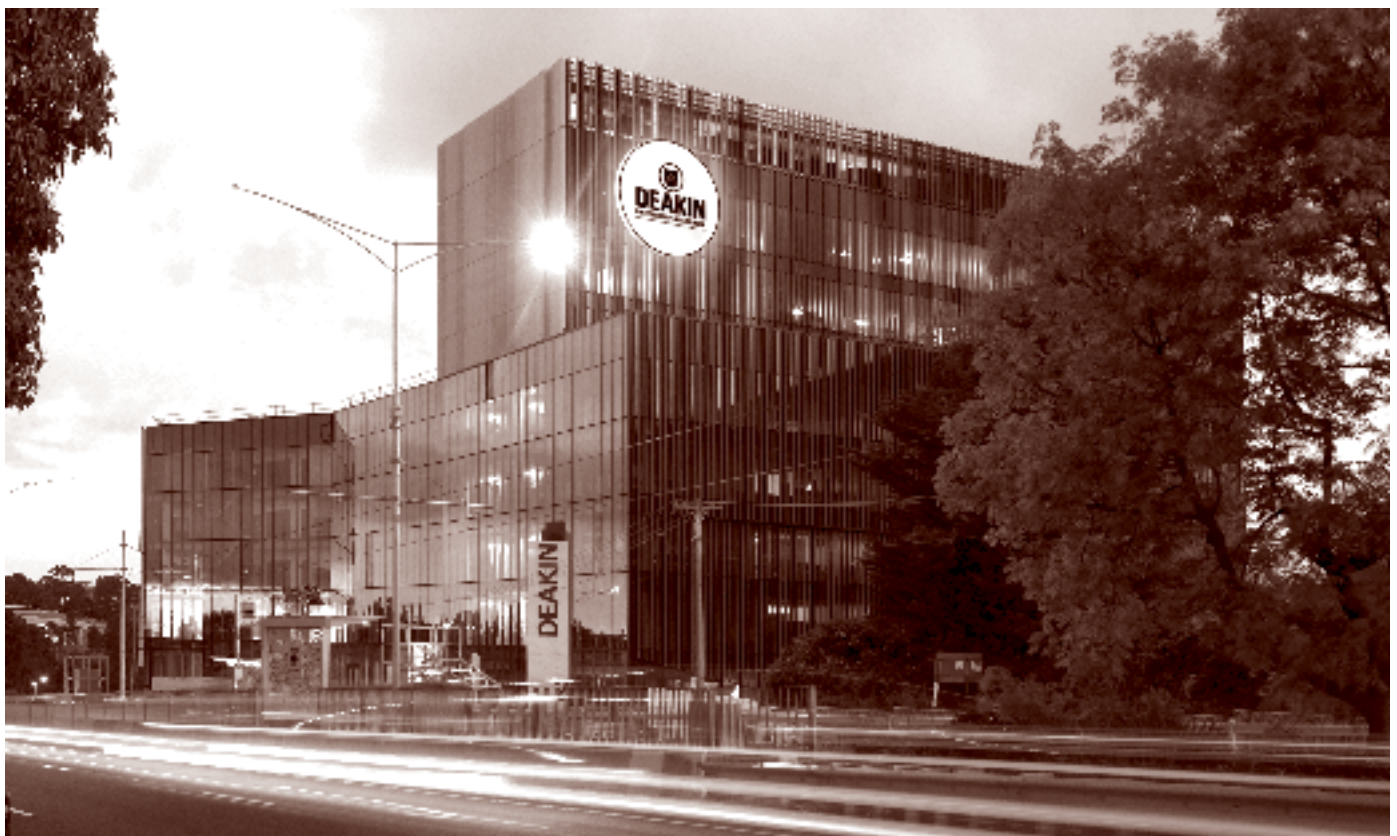
Burwood Highway frontage building.
