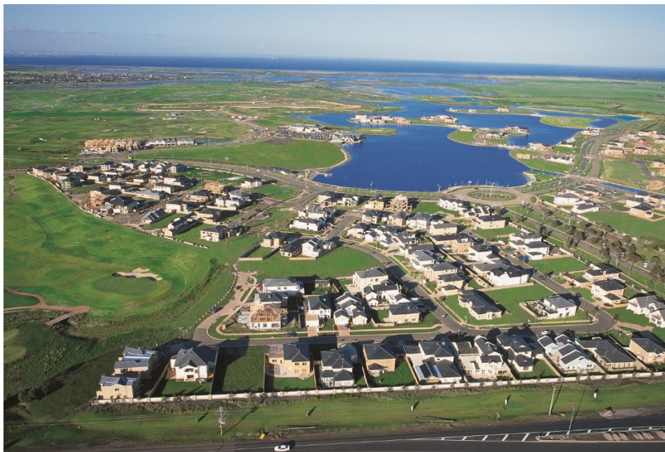
Figure 64: Sanctuary Lakes Resort, c.2000 Golf Course and Housing construction underway. Photo: @Sanctuary Living
